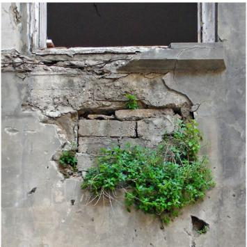
Plants like ivy cause similar damage because they cling to buildings by root systems that penetrate cracks between bricks.
