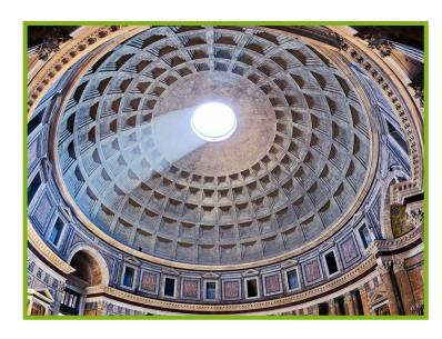
Roman concrete was different to the modern substance, but also very strong and durable. It was poured into molds in order to make the dome, which weighs 4,535 metric tons.
