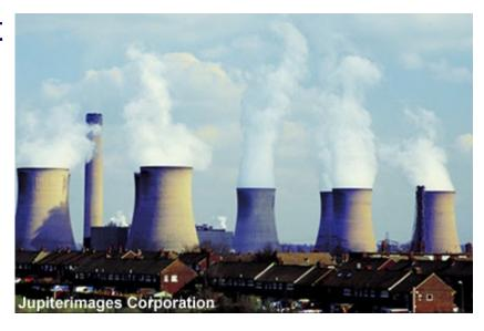
The cooling towers cool the steam, which condenses as water and can then be recycled in the power station.
